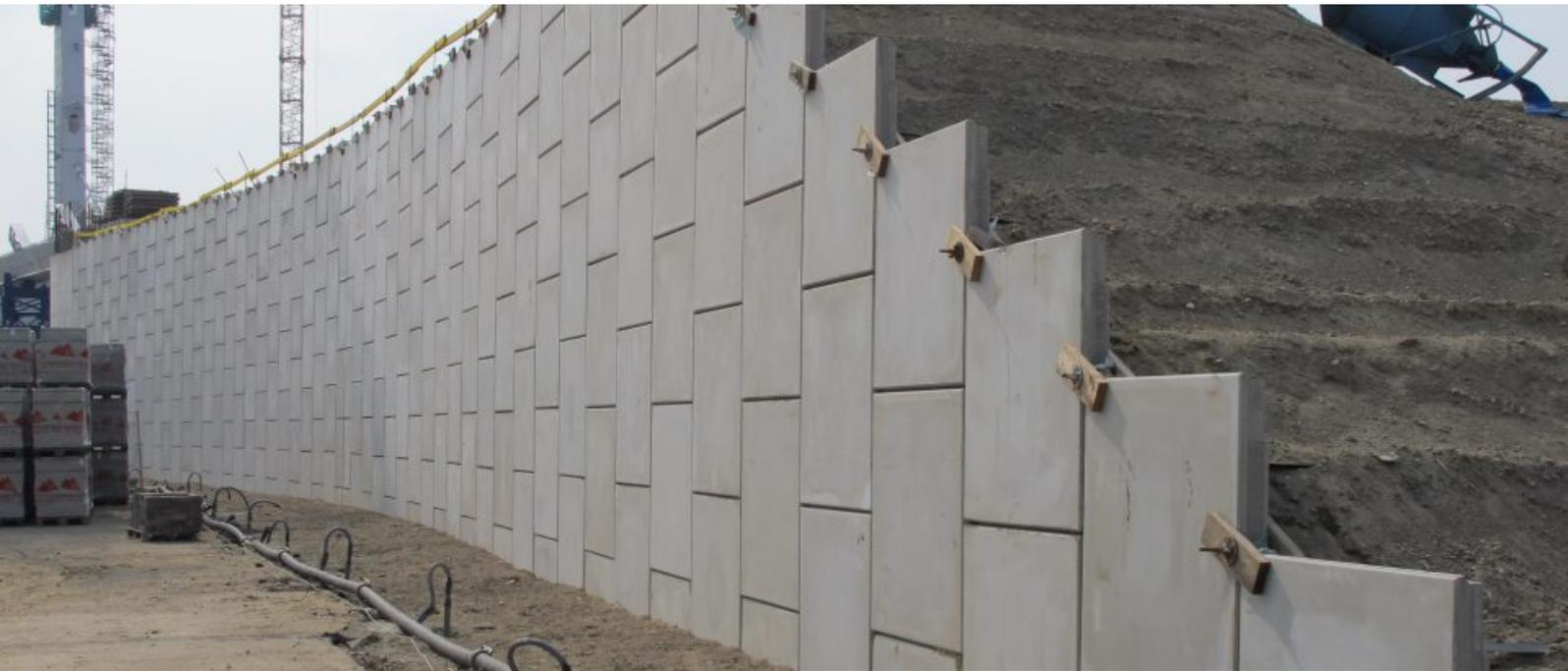
MURS DE SOUTÈNEMENT EN BÉTON AVEC BANDES D'ARMATURE
