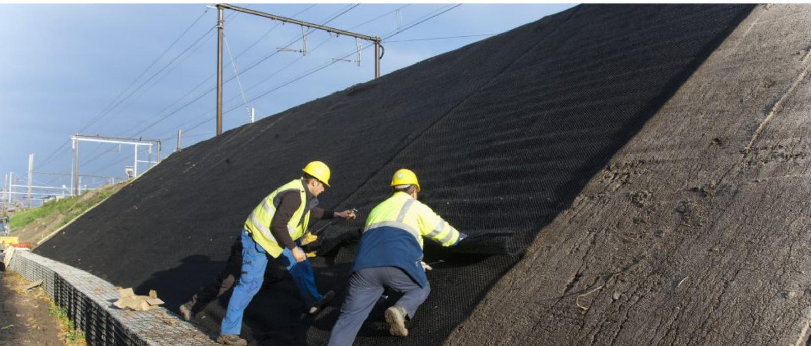
GÉOCOMPOSITE 3D, RENFORCÉ AVEC UNE ARMATURE EN ACIER OU EN POLYESTER
