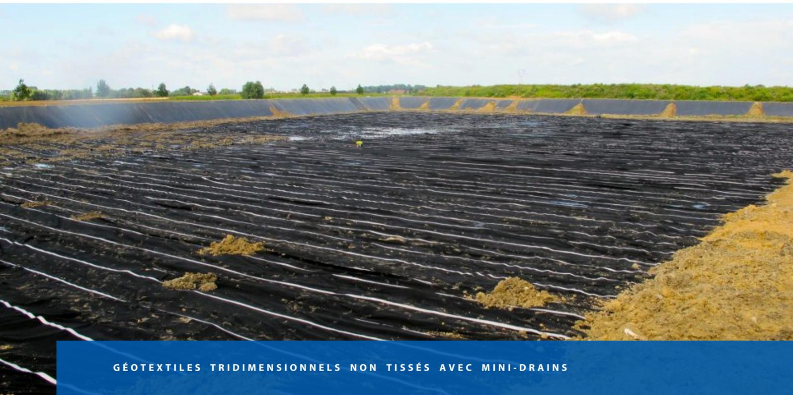
GÉOTEXTILES TRIDIMENSIONNELS NON TISSÉS AVEC MINI-DRAINS
